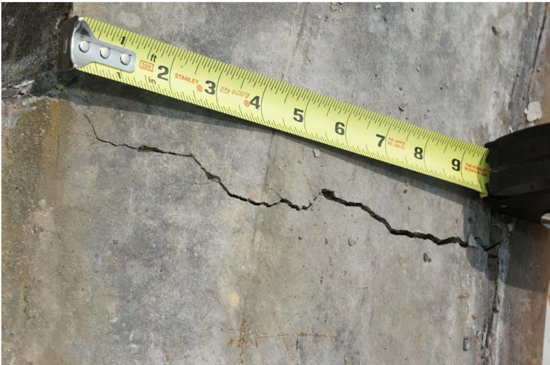
**Fig. 4. Crack in top surface of shielding wall adjacent to impacted buttress.**
