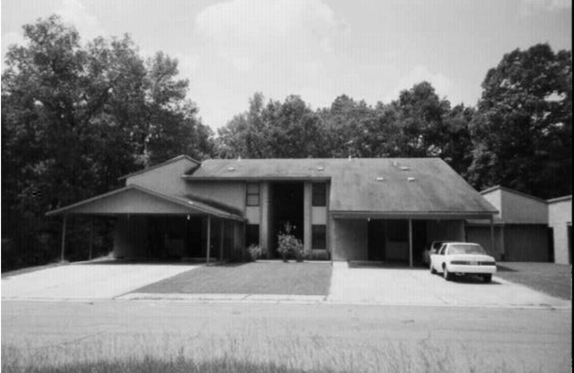
Figure 1.1: Fort Polk GHP residence (lower left apartment of a five-plex).
